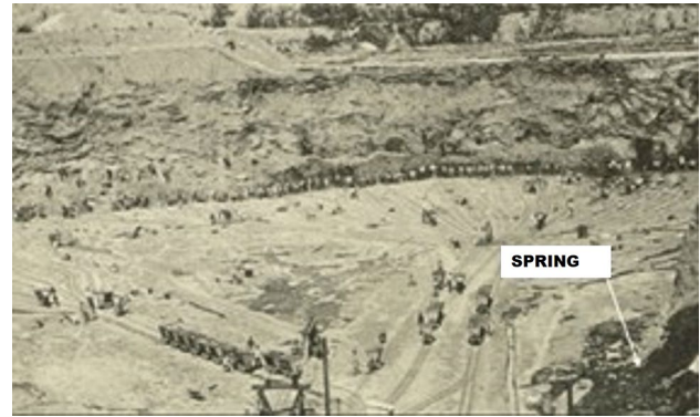
Fig. 4 Wesselton mine in 1896 with spring flowing at 220,000m 3 /d (Williams 1906)
